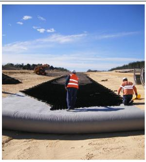
After consultation it was agreed that the innovative Geoweb® cellular confinement system would be an ideal solution for erosion protection of the swale drain and also provide soil stabilisation for the infill material.
